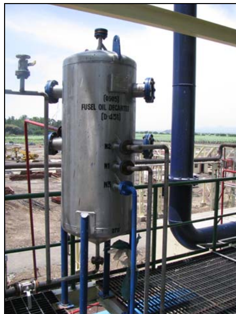
Figure 7: Metahara Distillery Rectifier Column and Fusel Oil Decanter
